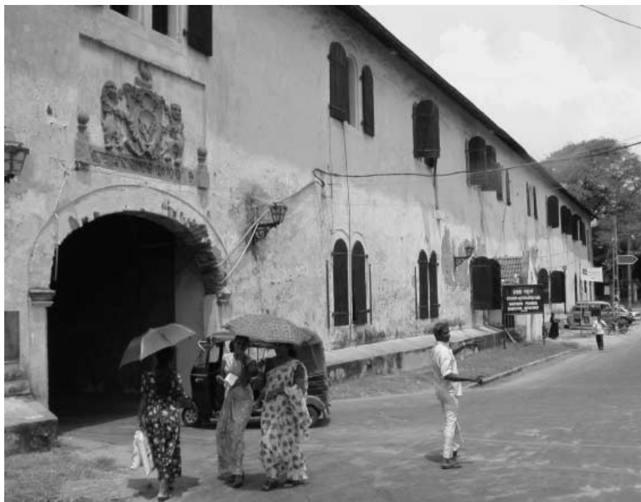
Figure 3. The VOC warehouse, built in the 1660s, played an important role in the logistics of the shipping and the trade. After restoration it will house the New Maritime Museum. (Avondster-Project)
