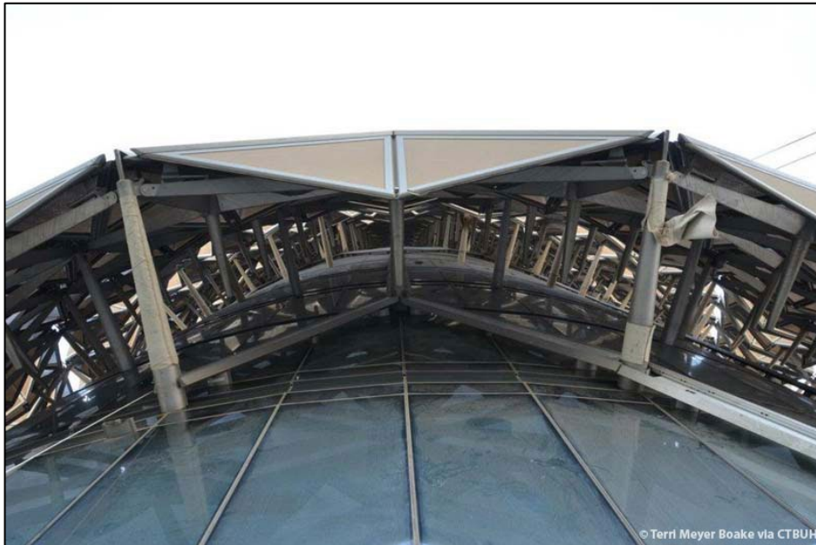
Figure 4: Image of the façade system's cantilever arms and brackets connecting to the main steel structure (Boake, n.d.)
