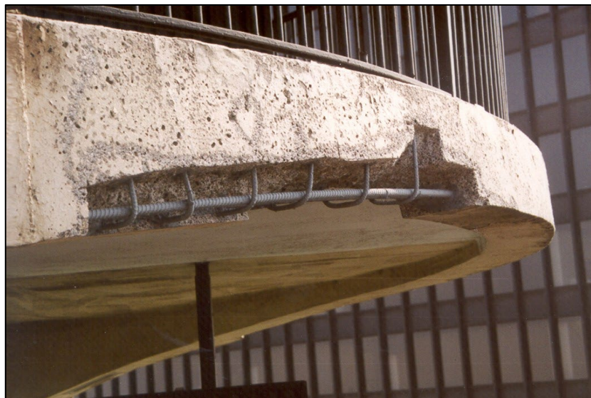
Figure 11: Image of concrete repair (WJE Projects, 2019).
