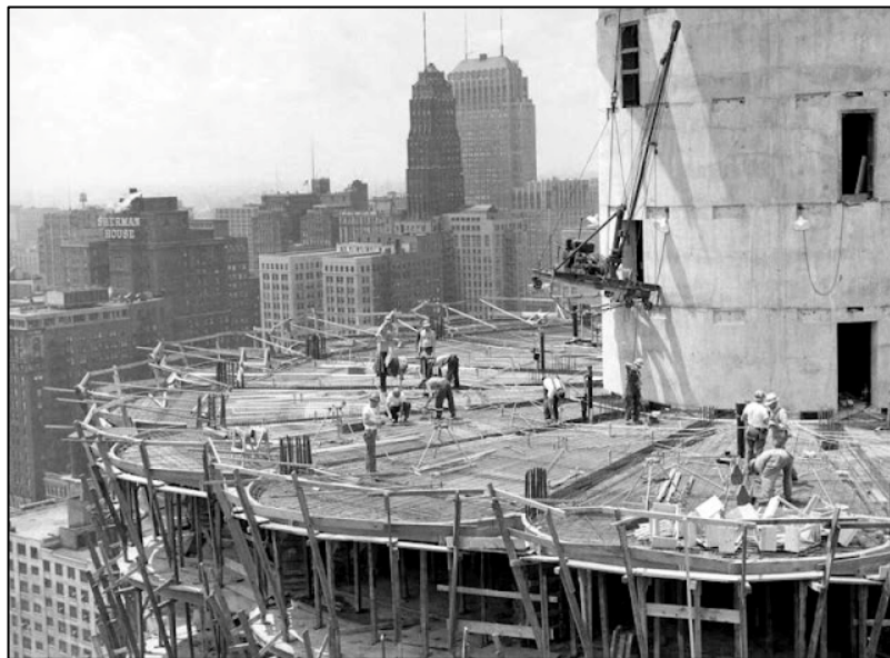
Figure 10: Image taken in 1961 during the construction of concrete being poured surrounding the concrete core (Chicago Old and New, 2019).
