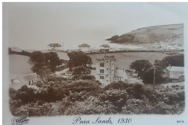
Plate 12) Pengersick Castle, restored, with new kitchen extension, c1930.
