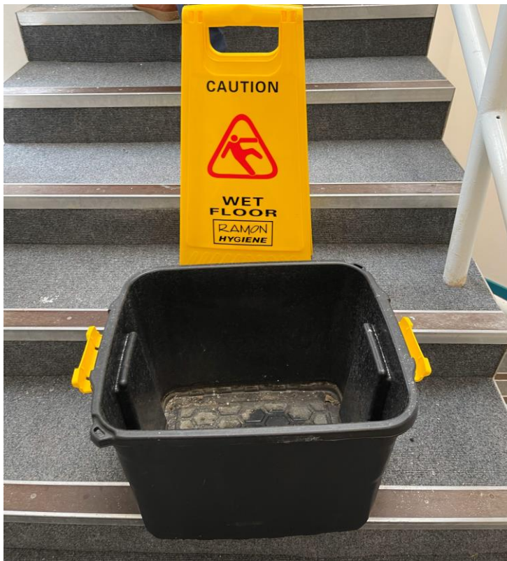
Photo showing container placed to collect water from the leaky cupola. (own image, 2024)
