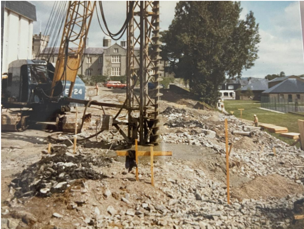
Photo Installing piles 1984 Library extension. (UA|OM|418)
