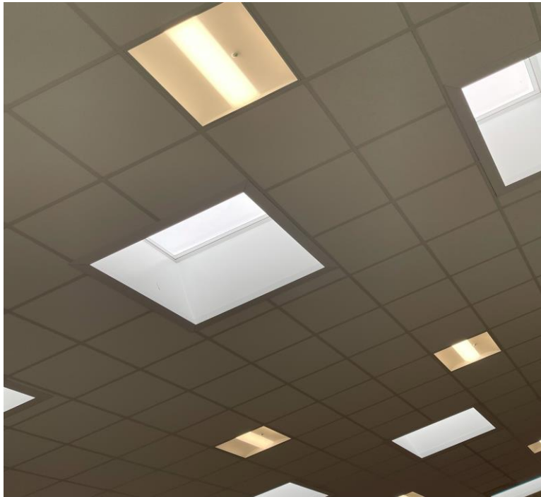
Photo showing roof light and lighting fixtures.
