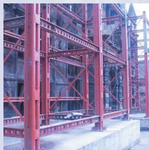
Botany Building, Glasgow Reigart Contracts Ltd
