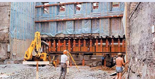
Falkirk, Scotland WJ & D Demolition
