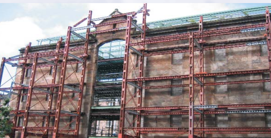
Fox Street, Glasgow Hunter Demolition
