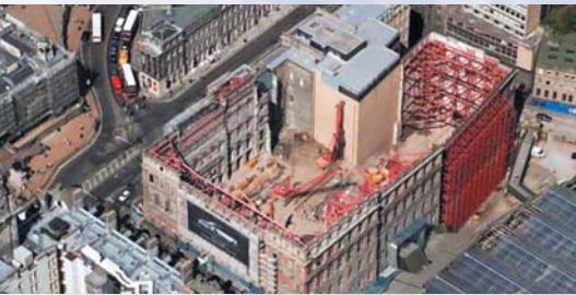
Waverley Gate, Edinburgh. Balfour Beatty Civil Engineering Ltd.
