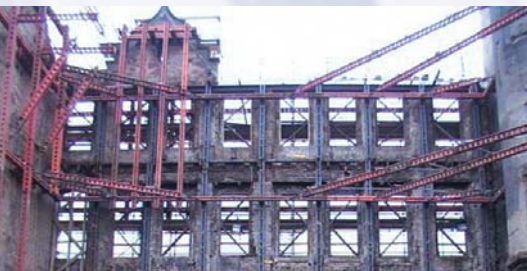
Rutherglen Town Hall Dem-Master Demolition Ltd
