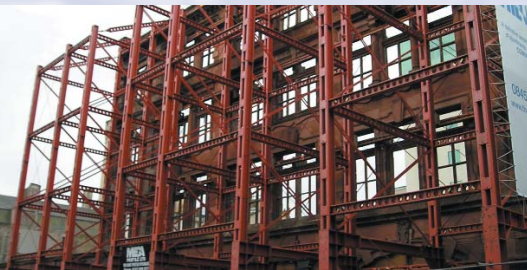
Oswald Street, Glasgow JCJ Demolition & Construction Ltd.
