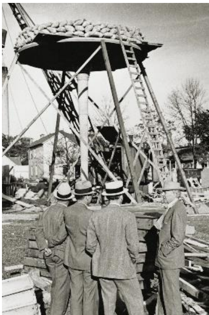
Figure 68: Testing the strength of the full-scale model of one of the columns designed for the SCJ headquarters. (Photo credit: S.C. Johnson & Son Inc.)
