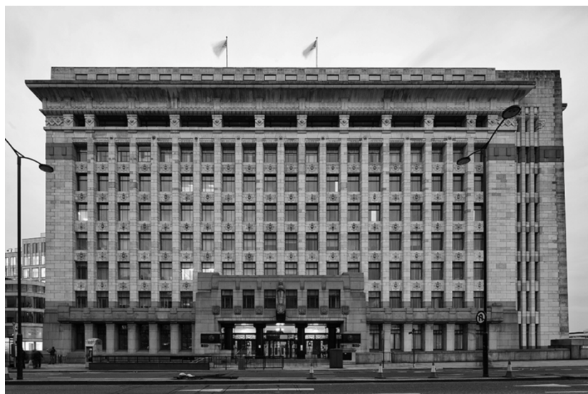
Figure 2: Adelaide House. (Photo by, David Bank)
