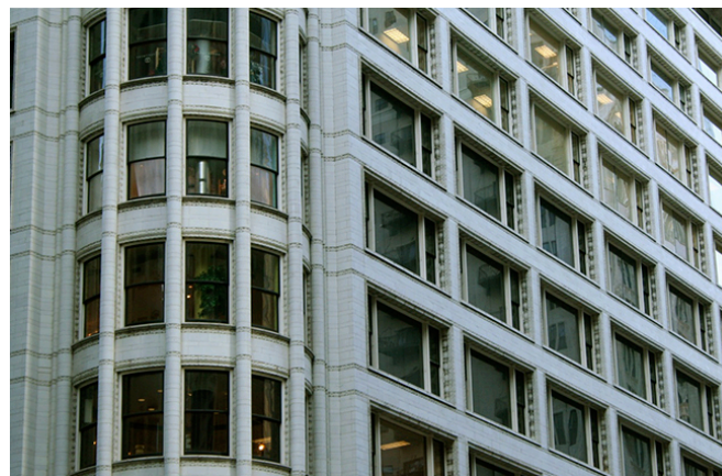
Figure 4: The Carson, Pirie, Scott and Company building demonstrating the Chicago windows. (Photo by, Kevin Zolkiewicz)
