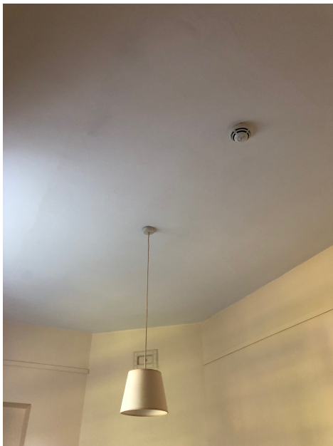
Figure 1: Example of Halogen Lighting
