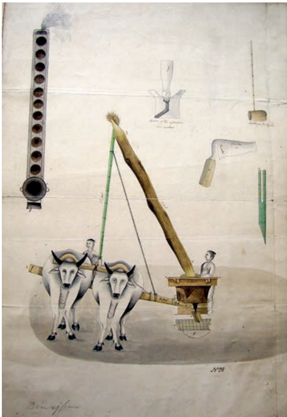
Plate 12.11 A sugar mill operated by oxen. Commissioned by Francis Buchanan during the Survey of Dinajpur, 1807–1808. British Library Private Papers, Mss Eur G25, f. 25.
