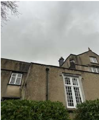
Figure 2 - Showing exterior traditional windows with metal transom topped by gothic style arched heads. This figure also shows detailed stone surround and the potential modern cement base.
