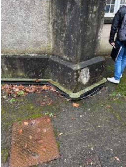
Figure 4 Showing loose wiring on the external grounds around building also featuring the buildings cut stone footings
