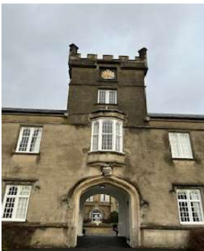
Figure 3- displaying a Tudor arch with an ornate figure positioned in the middle above the opening. Also showing the decorative turret.
