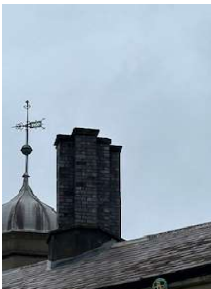
Figure 6 Showing traditional slate roofing materials along with the traditional round turret made from lead and topped with a decorative spindle and its original brick chimney stack
