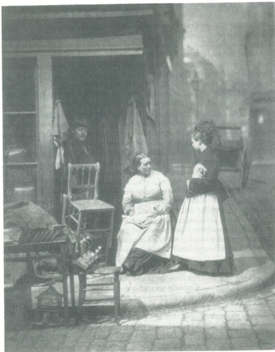
Plate 3.3 Second-hand furniture shop, Church Lane 1877 (just prior to demolition), John Thomson
