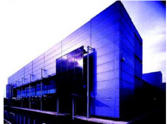
Baglan Energy Park industrial building
