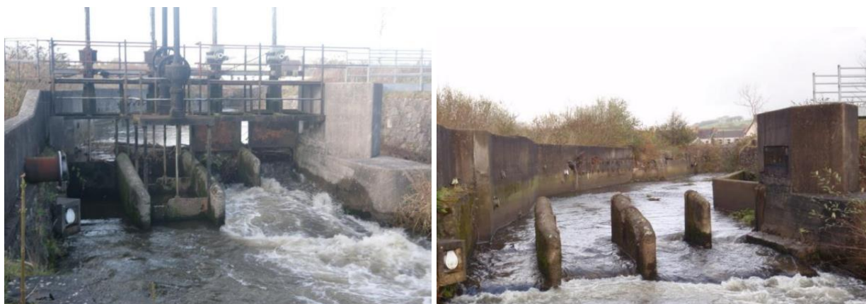
Figure 10 and 11: Afon Taf fish passage improvement project 2011
