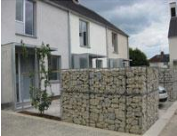
The Triangle, Swindon, hemcrete and timber frame
