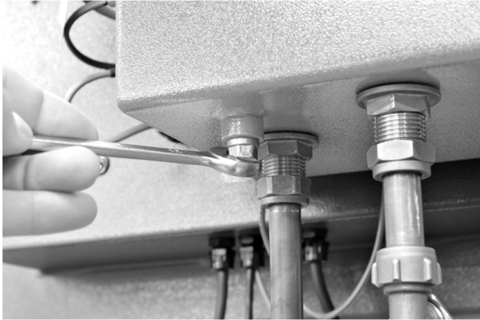
Figure 58 To Drain the Heater Tank
