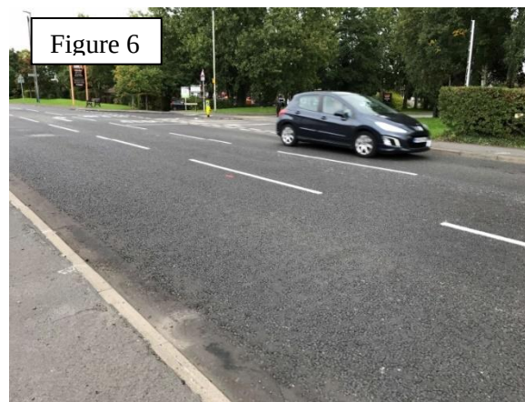
Figure 5 & 6 – Photos of the A7 in Carlisle of newly laid asphalt that incorporates MacReburs MR6 product.
