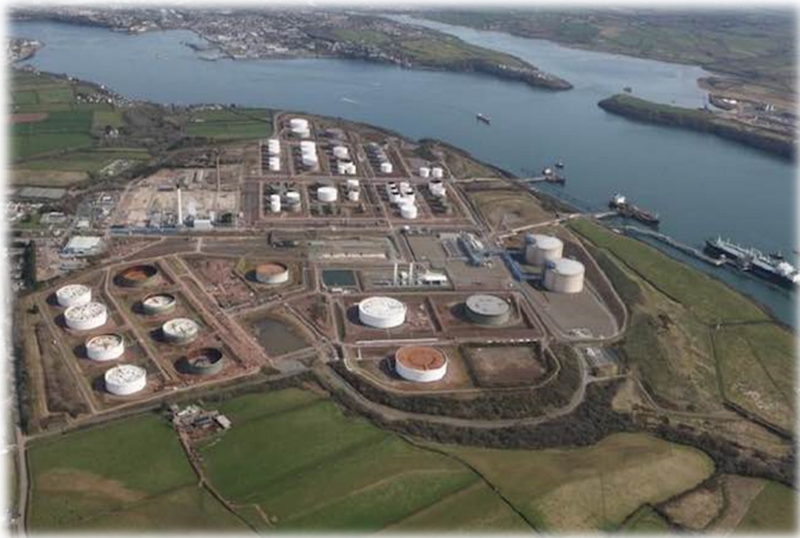
Figure 1 – Sem Logistics Milford Haven
