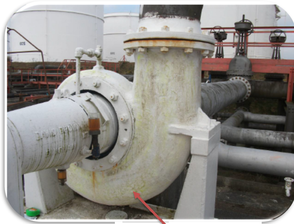
Point measured at 6.6mm thickness
