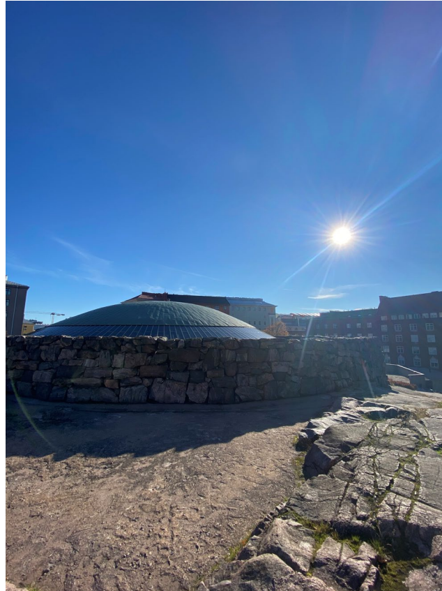
Figure 18: View of the 24m diameter dome (Photo credit: A. Messer)
