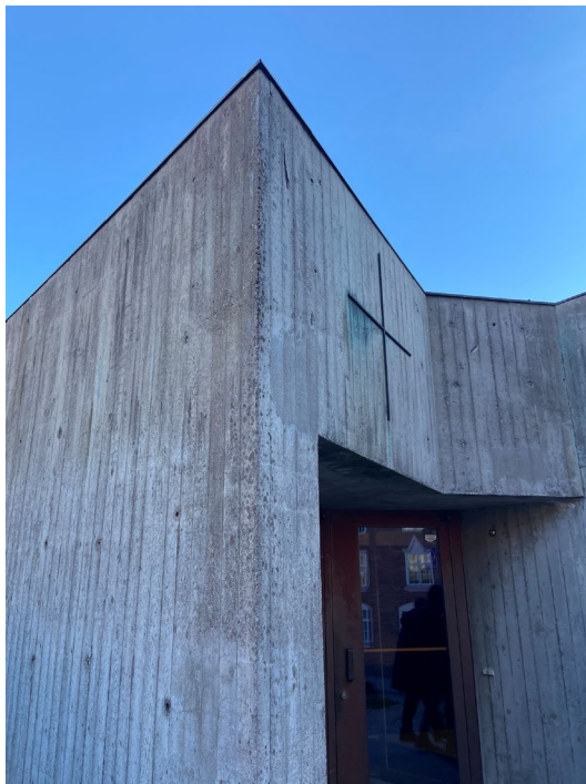
Figure 14: Timber pressed concrete walls with subtle cross symbolism (Photo credit: A. Messer)
