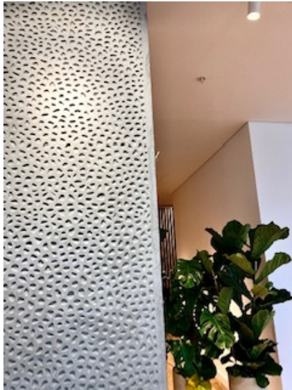
Figure 17: Cast patterns of the trabecular system on the concrete columns (Author , 2021)
