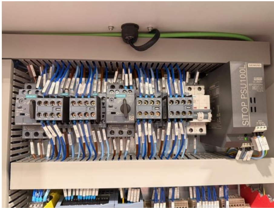
Figure 6 - Power supply and circuit/overload protection.
