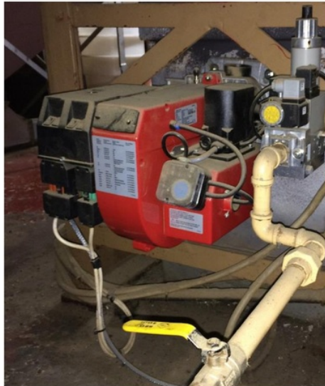
Figure 5: The gas system including the solenoid and ignitor connected to the roasting drum.
