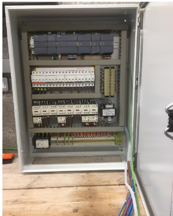
Figure 50: Shows the completed back plate fixed into the panel.
