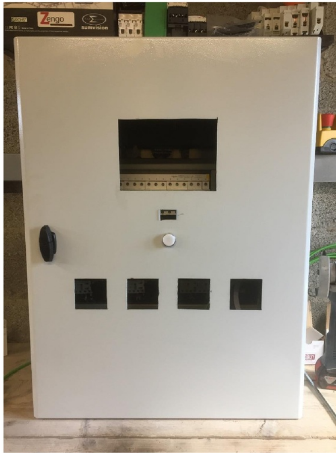
Figure 51: Shows the result of the holes being made for the door elements of the project.
