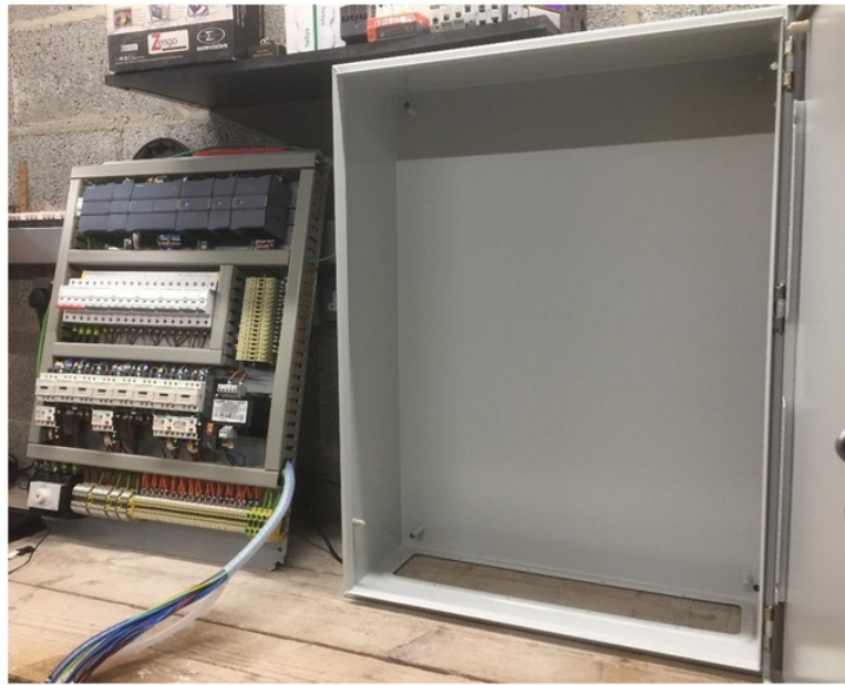
Figure 49: Shows the completion of the back plate.
