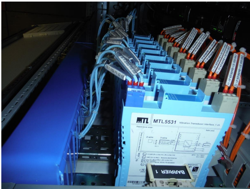
Figure 4, source: H Raymond. Example of barriers used between the sensing element and PLC input card
