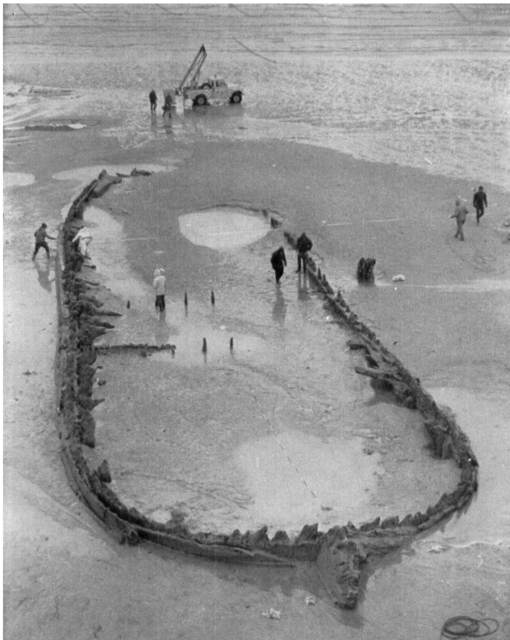
Figure 8 View of Amsterdam looking aft, showing the transverse partitions, and just outside the ship the end of the mast.
