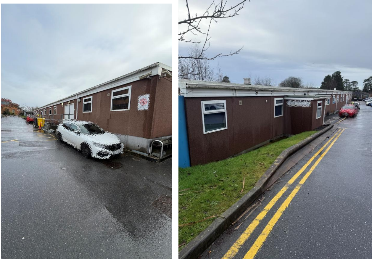
Figure 10 - Building J Exterior a. North-West Side b. North-East Side
