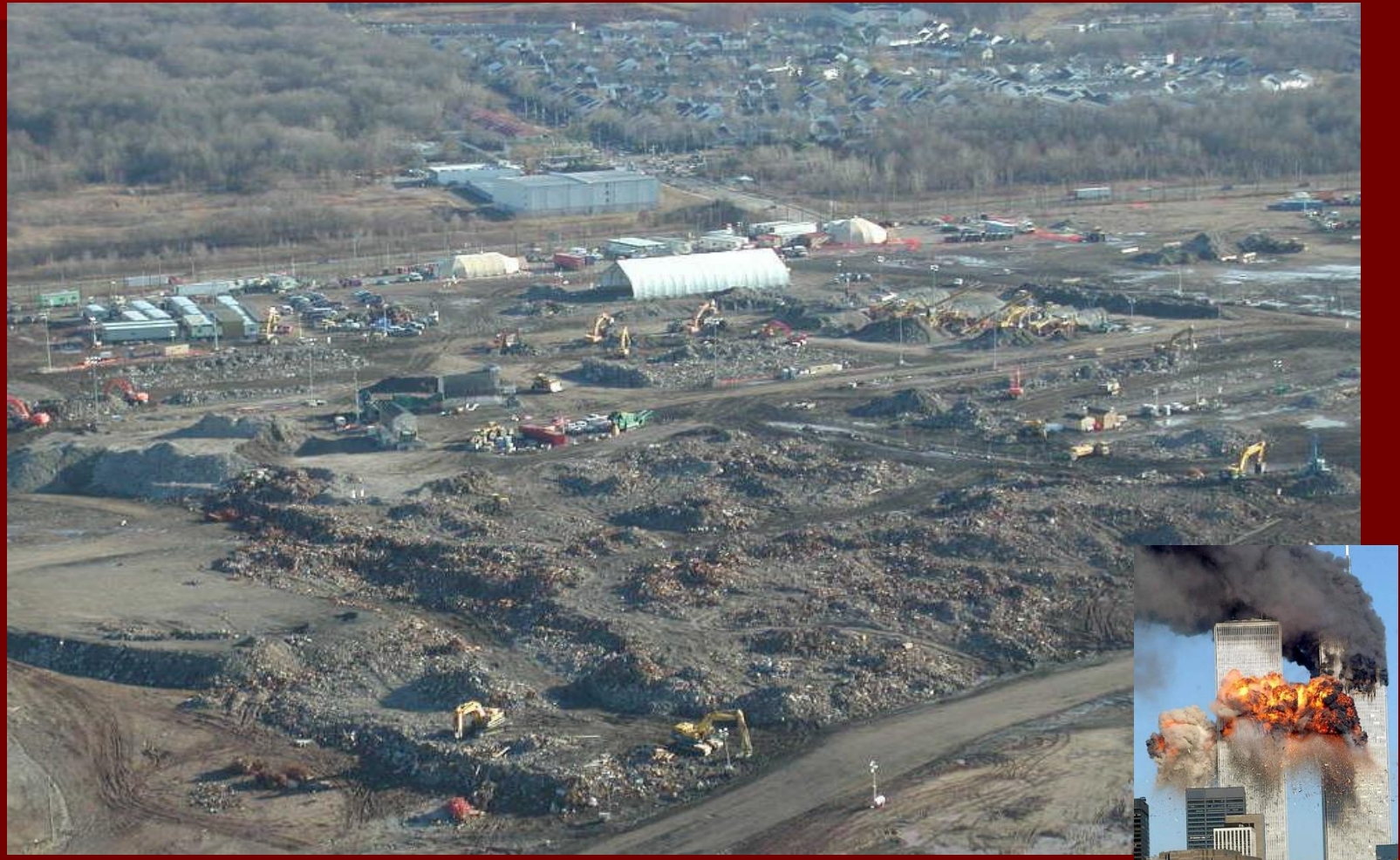
World Trade Center debris is stored in view of residential neighborhood (Brown, 2004)
