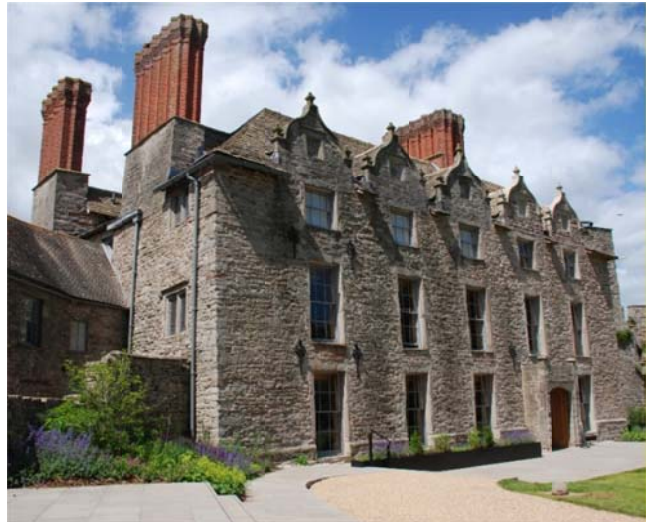
Figure 48: Hay Castle House, Hay-on-Wye (image credit: breconbeacons.org).
