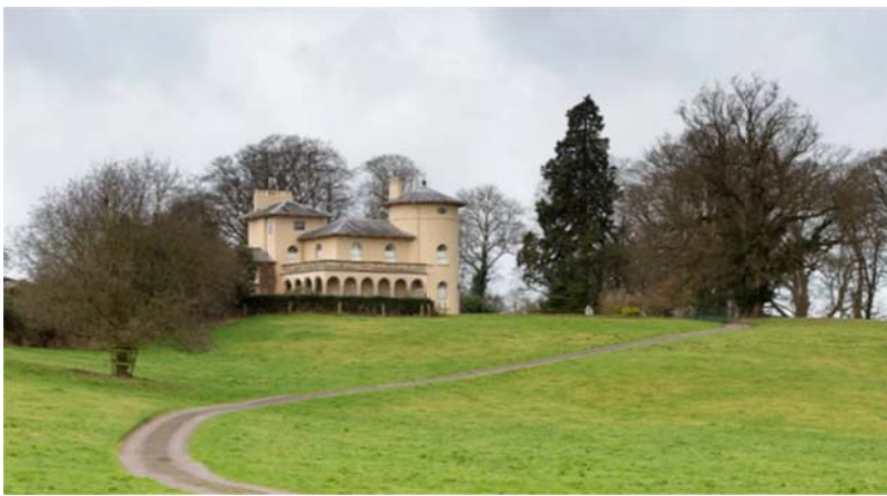
Figure 35: Restoration project returned Cronkill to its original colour (image credit: National Trust).
