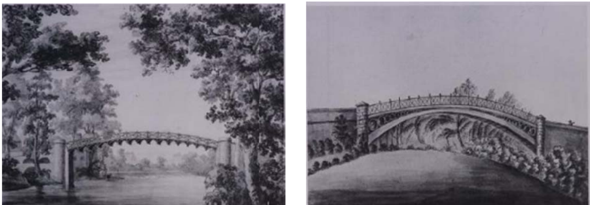
Figure 25: Original and replacement iron bridges at Stanford-on-Teme (image credit: Michael Mansbridge).
