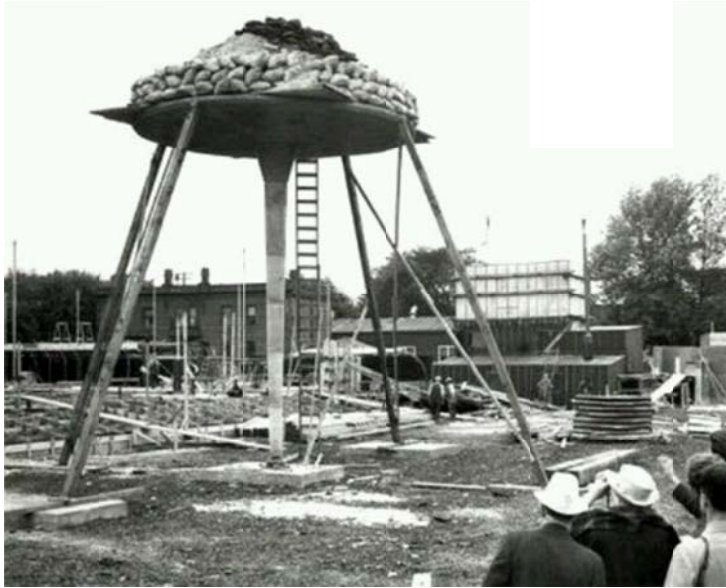
Figure 31: Testing the lily-pad columns (image credit: Pinterest).
