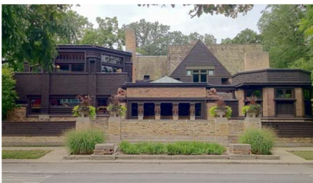
Figure 49: Oak Park, Wright's home and studio 138 (image credit: Frank Lloyd Wright Foundation).
