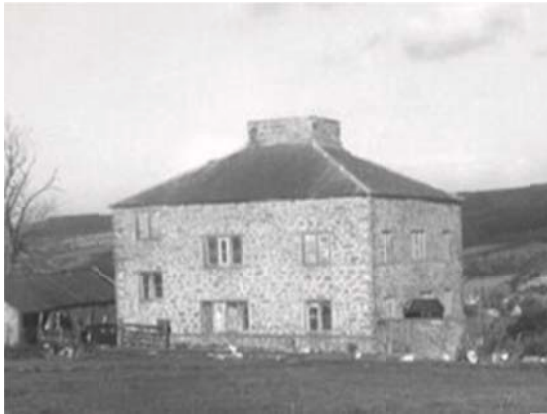
Figure 56: Trimley Hall, Flintshire (image credit: Coflein).
