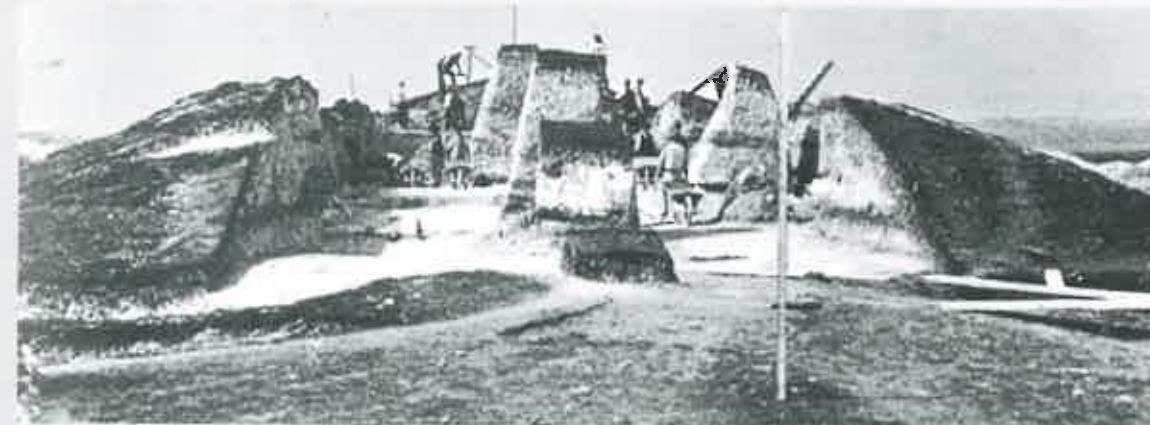
Excavation in progress at Wor Barrow, Cranborne Chase (above). The barrow was eventually removed
