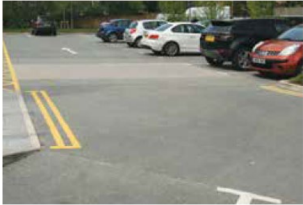
c Porous concrete
