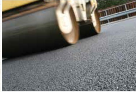
b Porous asphalt
