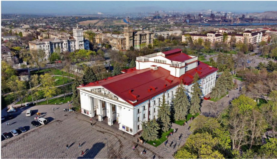
Figure 2-1 - Mariupol Drama Theatre Before 16th March 2022 [4]
