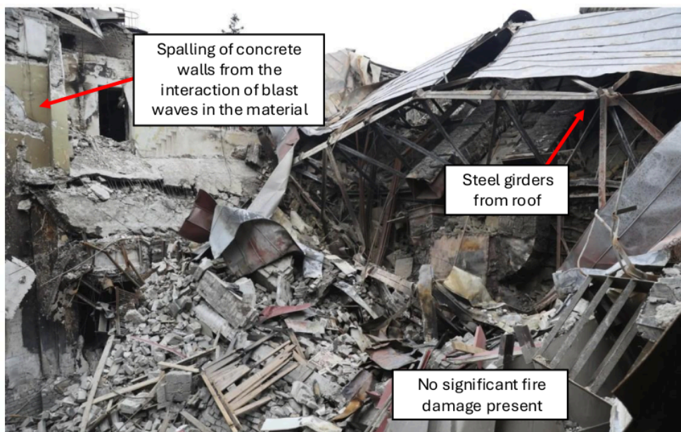
Figure 3-3 - Internal Destruction of Mariupol Drama Theatre [6] Highlighting Blast Damage and Lack of Significant Fire Damage
