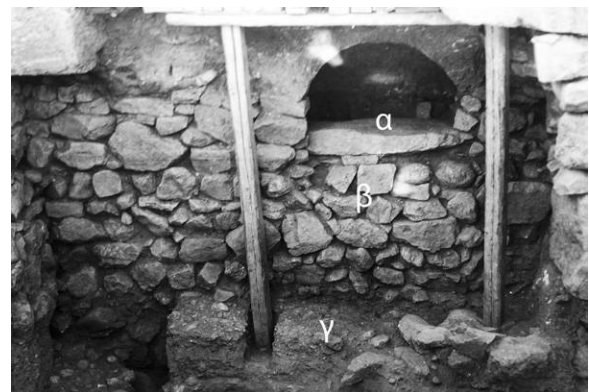
Fig. 14. Doorway to Room B3 from Room B1, seen from the east, showing the threshold (α), the foundation of Wall 11 (β), and the underlying Middle Helladic floor (γ). Notice the tunnel above the threshold, which was used by the excavators to access Room B3 (courtesy Archaeological Society at Athens, Photo Archive, A/A 1281).
