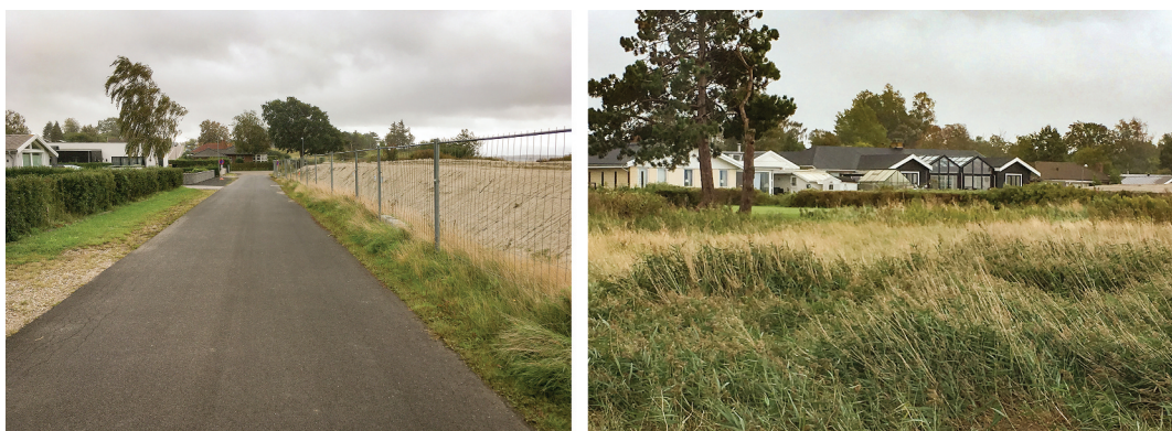
Figure 5. Houses still facing the salt meadow and houses now facing the 2.4 metre dike towards the fjord at Jyllinge Nordmark. Both photos from August 2020. Photo: Gertrud Jørgensen.
