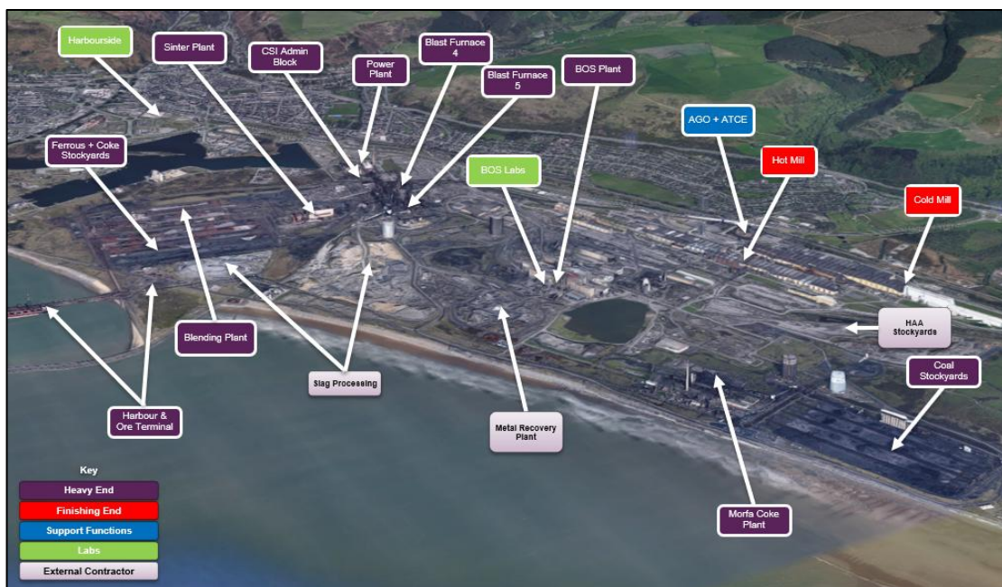
Figure 4 - Ariel View of Port Talbot Steelworks
