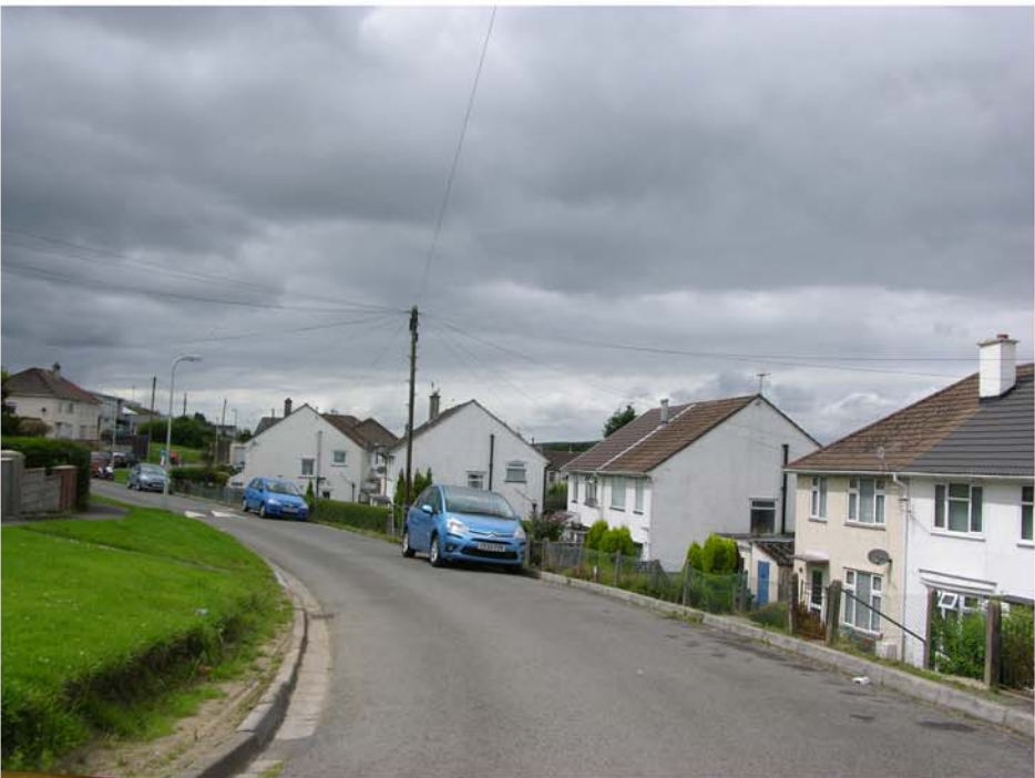
Examples of gable walls along Heol Caradoc.
