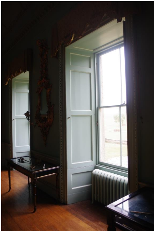
Fig 112 Room 9: Drawing Room showing panelled window reveals.
