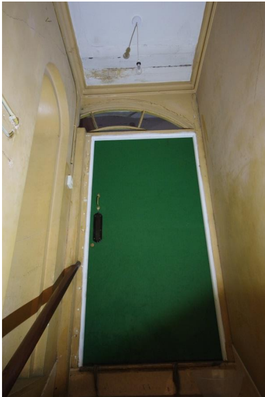
Fig 42 Room 1: Door at the top of the stairs and arched recess in the south wall.
