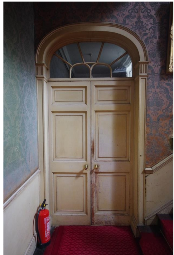
Fig 77 Room 6: Main staircase, door in west wall.
