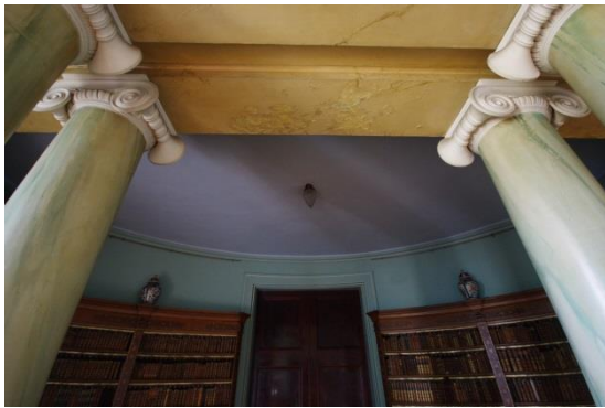
Fig 128 Room 9: Drawing Room, ceiling in apse end.
