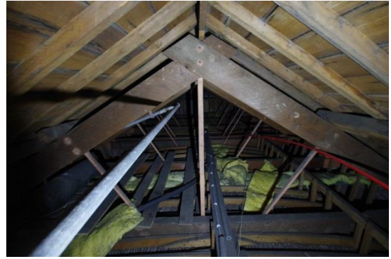
Fig 173 Roof structure above Drawing Room.
