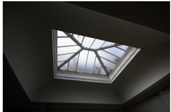
Fig 136 Room 10: First Floor Corridor, lantern above light well.
