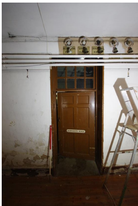
Fig 53 Room 3: South wall, door to the Servants' Hall.
