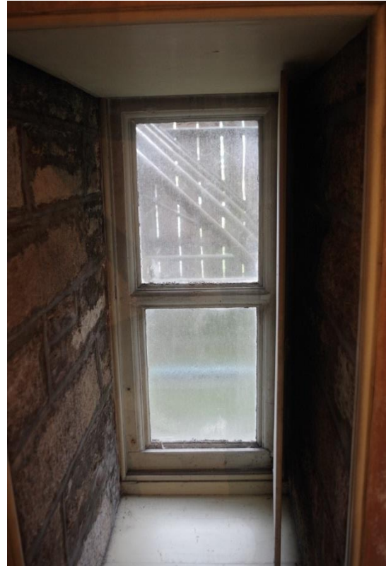
Fig 66 Room 5: China Closet, 18 th century window to east of front door.
