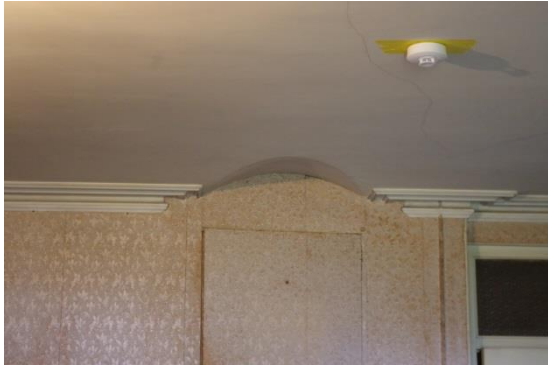
Fig 62 Room 4: House Keeper's Room, raised ceiling above the lancet window.
