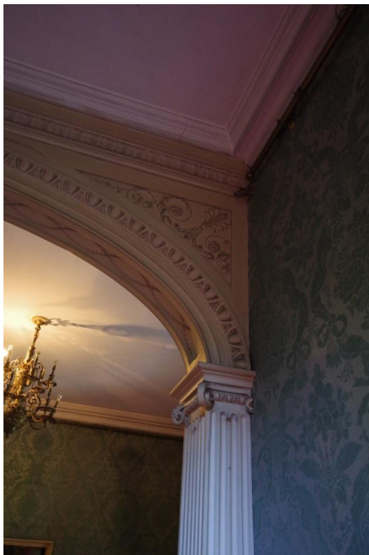
Fig 75 Room 6: Main staircase hall, detail of segmental arch to the east of the Main Staircase.
