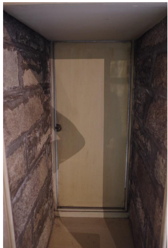
Fig 67 Room 5: China Closet, window shutter.
