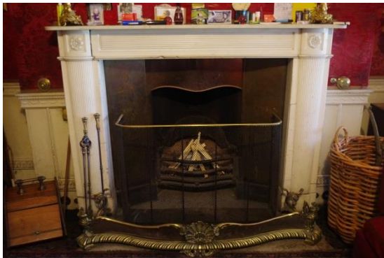
Fig 86 Room 7: Fireplace in the Morning Room, possibly by Soane.
