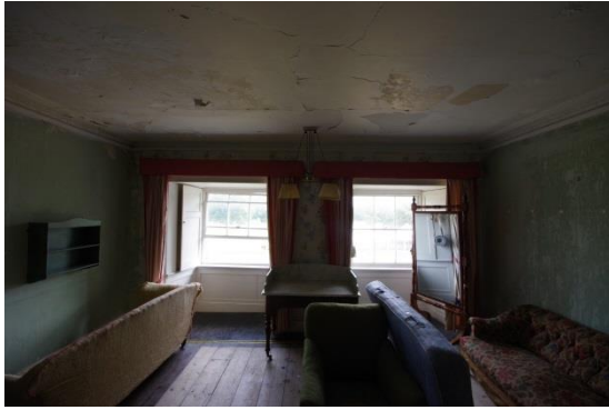
Fig 138 Room 11: Pink Bedroom, north wall.
