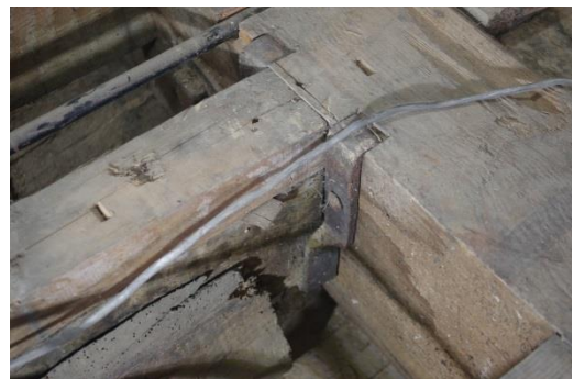
Fig 187 Room 11: Detail of Phase 2 beam with a joist hanger supporting a Phase 1 joist (with strip of timber on top to make up floor height).
