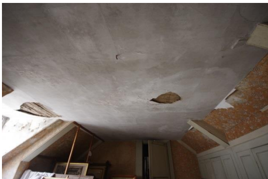
Fig 171 Room 15: Attic Gable Room ceiling.
