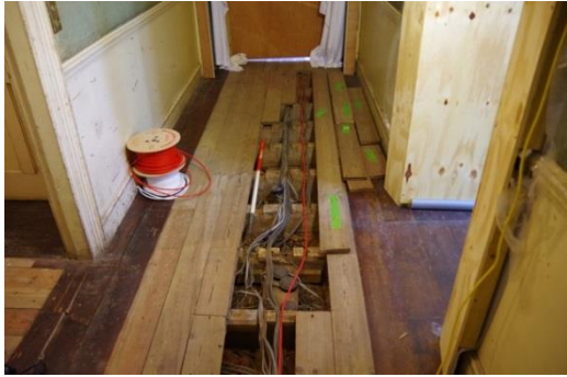
Fig 181 Room 10: Opened floor in First Floor Corridor looking west.
