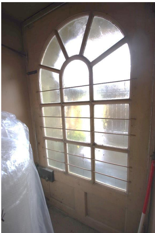
Fig 34 Room 1: detail of entrance door in north wall.
