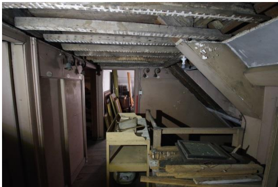
Fig 164 Room 14: Attic Landing looking south.
