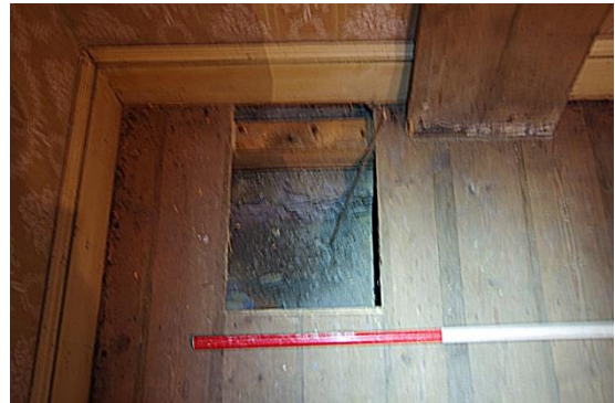
Fig 177 Room 5: Opening in the north-west corner of the China Closet.
