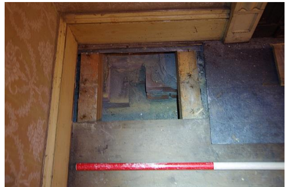
Fig 178 Room 5: Opening in the north-east corner of the China Closet.
