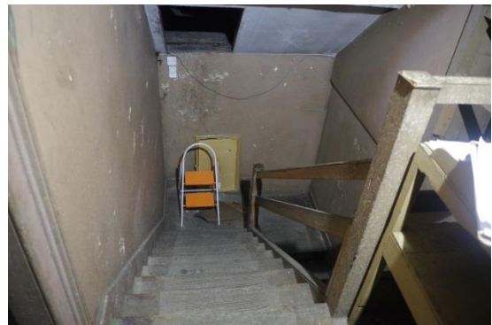
Fig 161 Room 14: Attic stairs, looking west.
