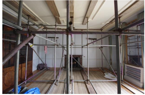
Fig 99 Room 8: Saloon, west wall.
