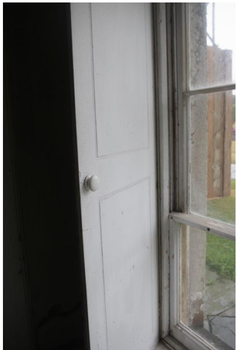
Fig 58 Room 4: House Keeper's Room, window shutter.
