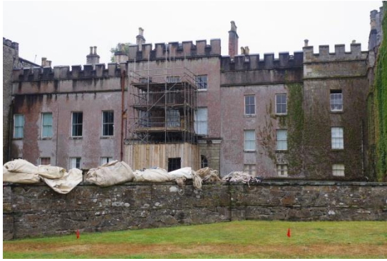
Fig 25 North elevation of main east-west range.
