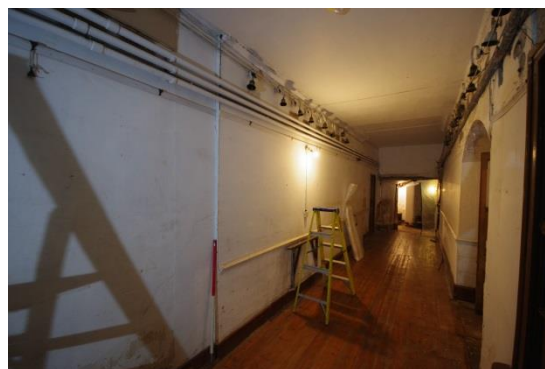
Fig 54 Room 3: View of the south wall looking west.
