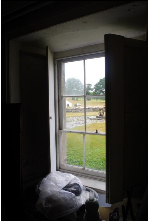
Fig 57 Room 4: House Keeper's Room, six over three sash window in north wall.
