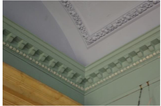
Fig 124 Room 9: Drawing Room, cornice.
