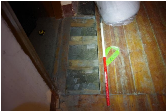
Fig 174 Room 3: Opening in the floor of the Basement Corridor abutting entrance to Housekeeper's Room.
