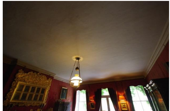
Fig 90 Room 7: Morning Room ceiling.
