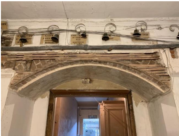
Fig 175 Room 3: Arch of door to Former Entrance Hall showing exposed brick arch and laths (photo courtesy of Greg Kaminski).
