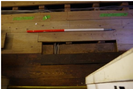
Fig 182 Room 10: Opened floor in First Floor Corridor with single plank lifted close to the door to the Blue Bedroom.
