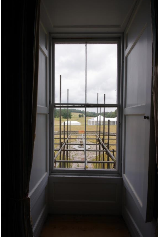
Fig 92 Room 8: Saloon, four-pane sash window in north wall.
