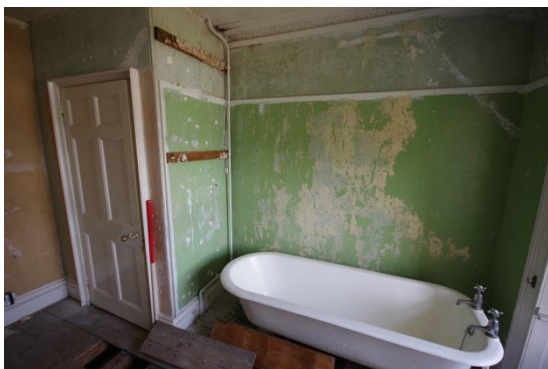
Fig 152 Room 12: Pink Bathroom, west wall.
