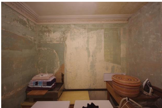
Fig 158 Room 13: Dark Room, west wall.
