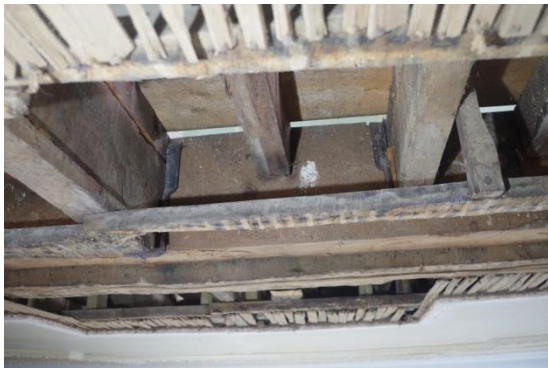
Fig 189 Room 11: Phase 1 and Phase 2 joists with Phase 2 beam and exposed Phase 2 ceiling structure of the Saloon.
