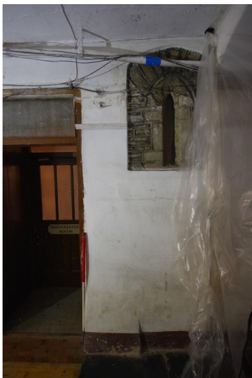
Fig 52 Room 3: North wall, door opening to the House Keeper's Room and a 13th century lancet window opening.
