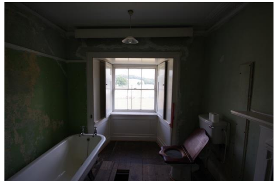
Fig 148 Room 12: Pink Bathroom, north wall.
