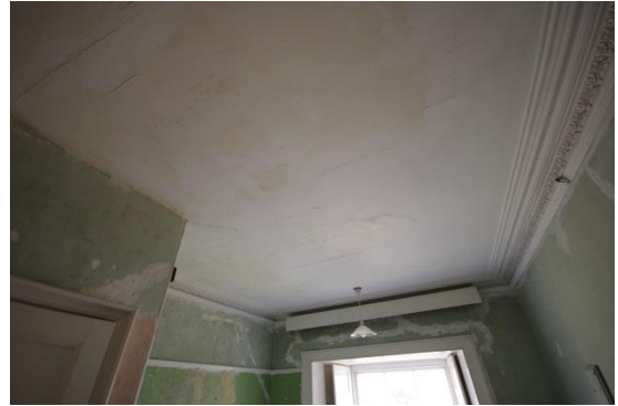
Fig 153 Room 12: Pink Bathroom, ceiling.
