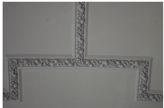
Fig 127 Room 9: Drawing Room, detail of ribs on ceiling.
