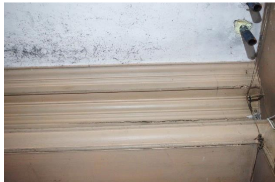
Fig 36 Room 1: Moulded cornice on north wall.
