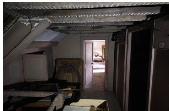
Fig 162 Room 14: Attic Landing looking north.
