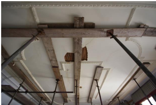
Fig 105 Room 8: Saloon, ceiling looking west.
