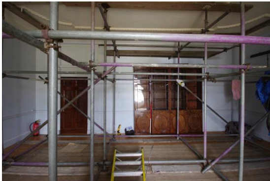
Fig 97 Room 8: Saloon looking south.
