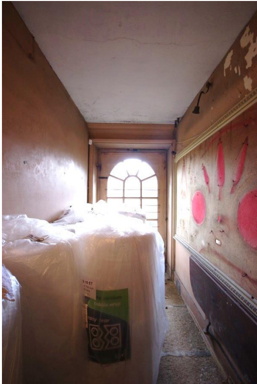
Fig 33 Room 1: Entrance door in north wall.
