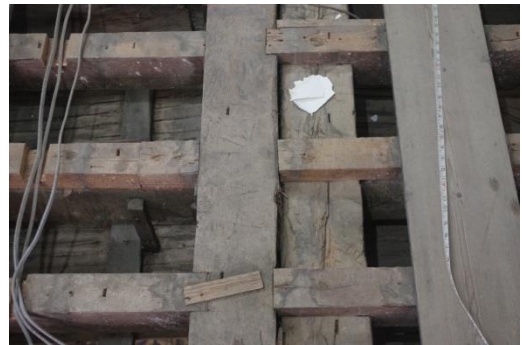
Fig 186 Room 11: Paired up floor beams: Phase 1 beam (right) and with Phase 2 beam (left) at slightly higher level.
