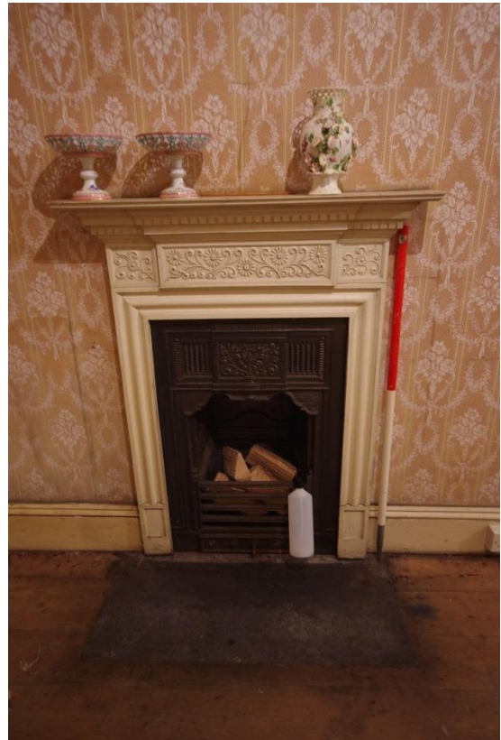
Fig 71 Room 5: China Closet, early 20th century cast iron fireplace in east wall.
