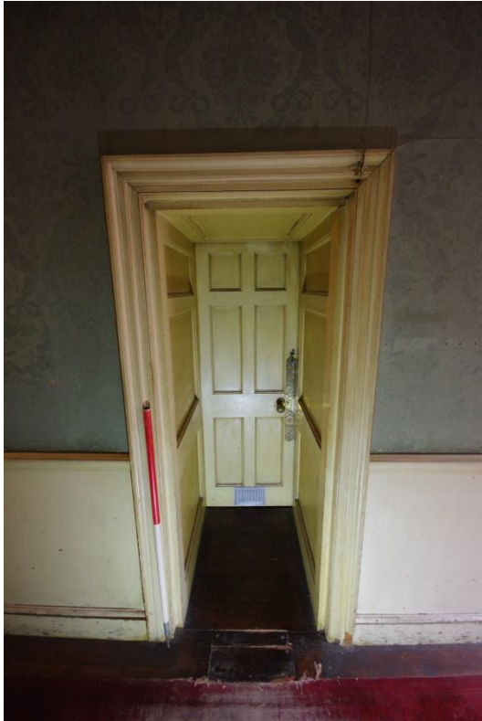
Fig 133 Room 10: First Floor Corridor, door to the Dark Room.
