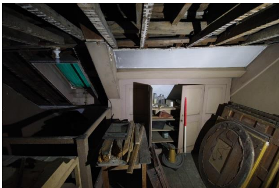
Fig 165 Room 14: Attic Landing looking west.
