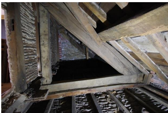
Fig 172 Roof structure to east of Attic Gable Room.
