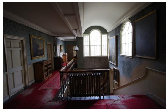
Fig 78 Room 6: Main Staircase, looking west at first floor.
