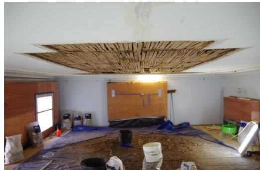
Fig 179 Room 8: The Saloon, showing the extent of the ceiling plaster removed (looking east).
