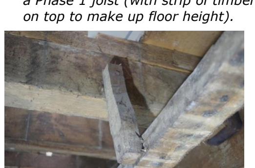
Fig 188 Room 11: Detail of phase 2 ceiling joist with vertical suspension batten.
