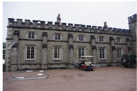
Fig 31 Service Wing, south elevation.
