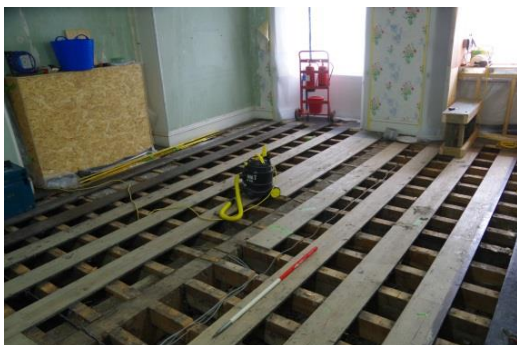
Fig 184 Room 11: looking north-west in the Pink Bedroom after the floorboards were lifted.
