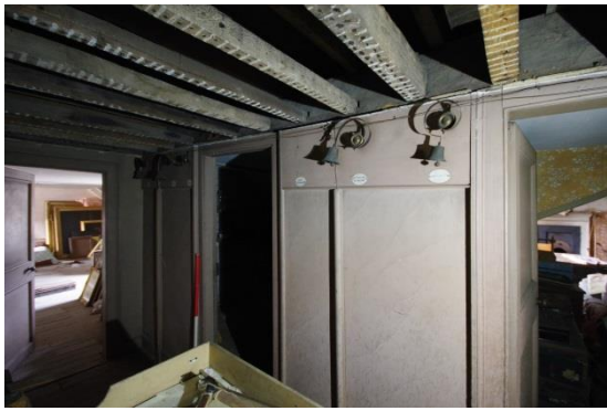
Fig 163 Room 14: Attic Landing east wall.
