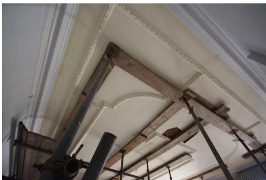
Fig 106 Room 8: Saloon, ceiling oblique view
