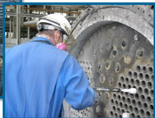
Figure 27: Tube side fouling (Parry, 2010)
