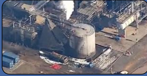
2011 Chevron Oil Refinery explosion, 4 dead
