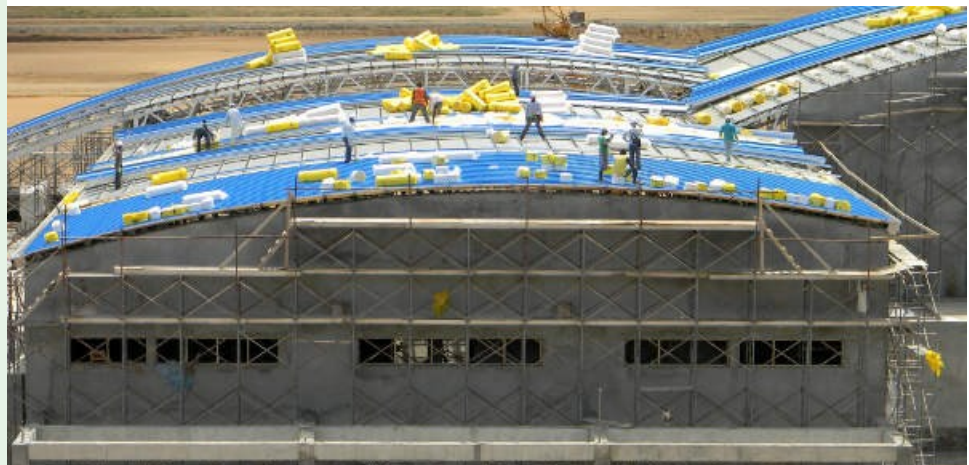
Image courtesy the Argyle International Airport Development Company Limited showing Traditional Construction Building Method in St. Vincent.
