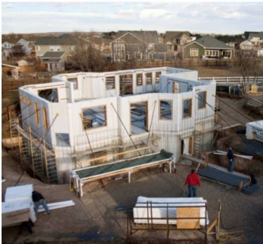
Home construction in USA using green building material, SCIPS (Photo by MotarSprayer.com)
