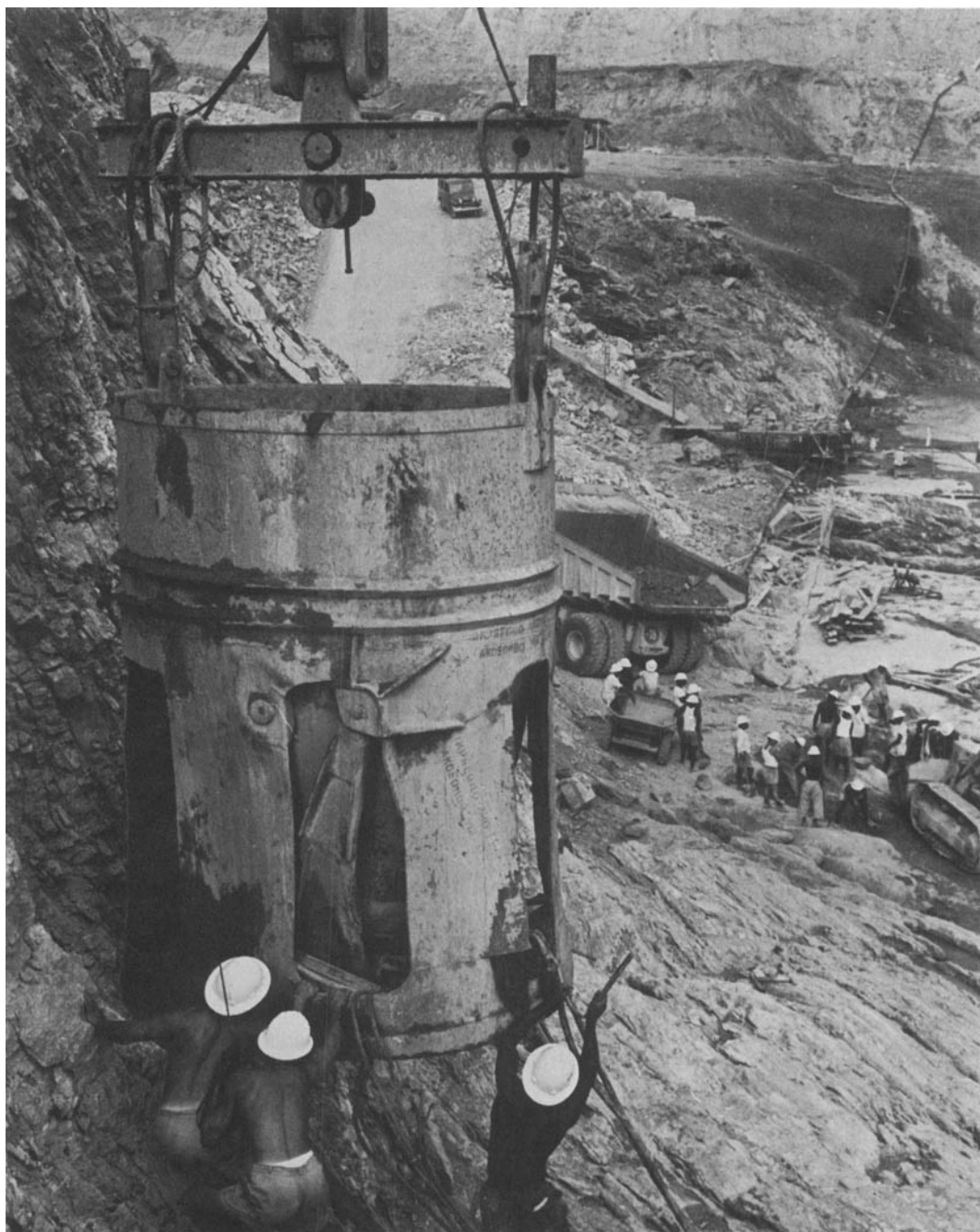
Work on the Volta Dam, Ghana.
