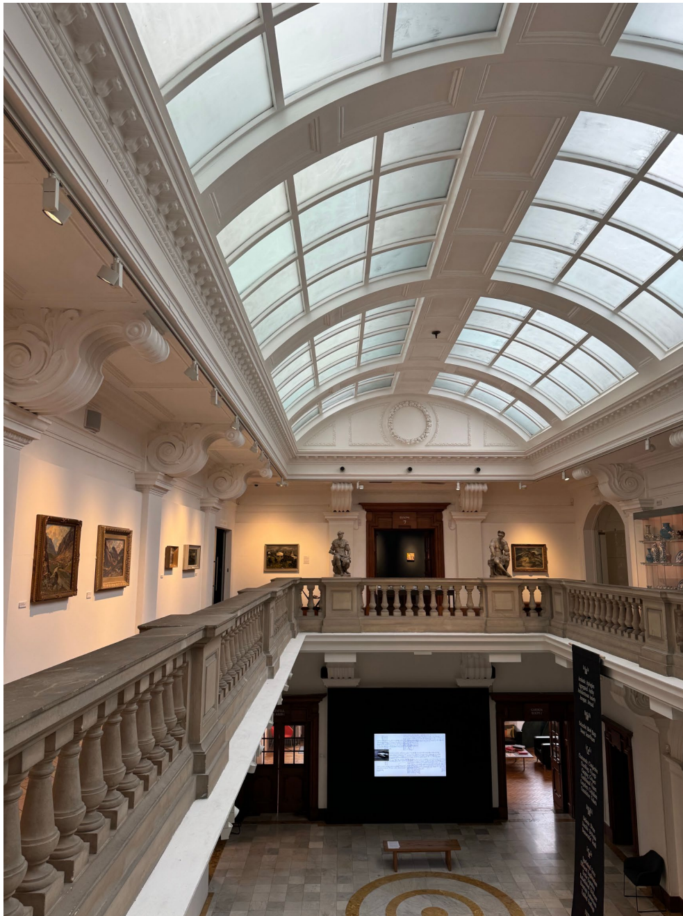
Figure 10: Rooflight above mezzanine level (Author's own, 2026).
