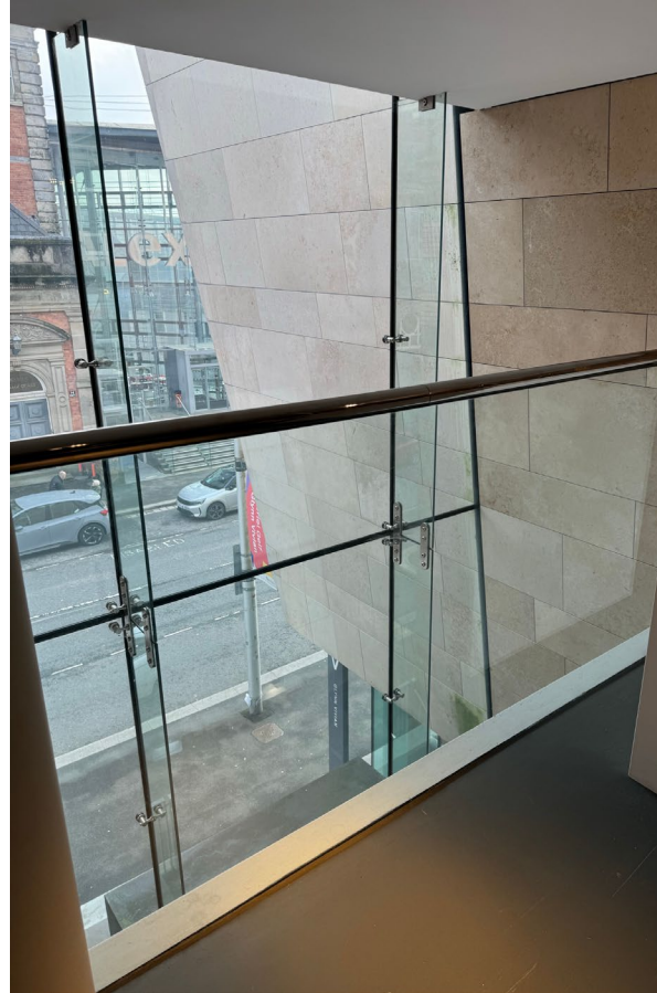
Figure 6: New curtain wall extension providing natural lighting (Author's own, 2026).
