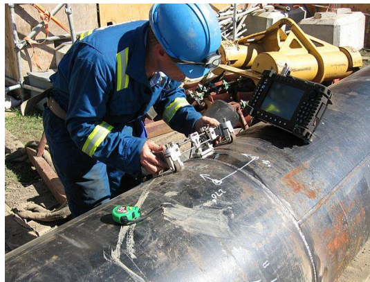
Figure 7 Ultrasonic Non-Destructive Testing - NDT - on Pipes using an ultrasonic flaw detector (sentin, 2020)
