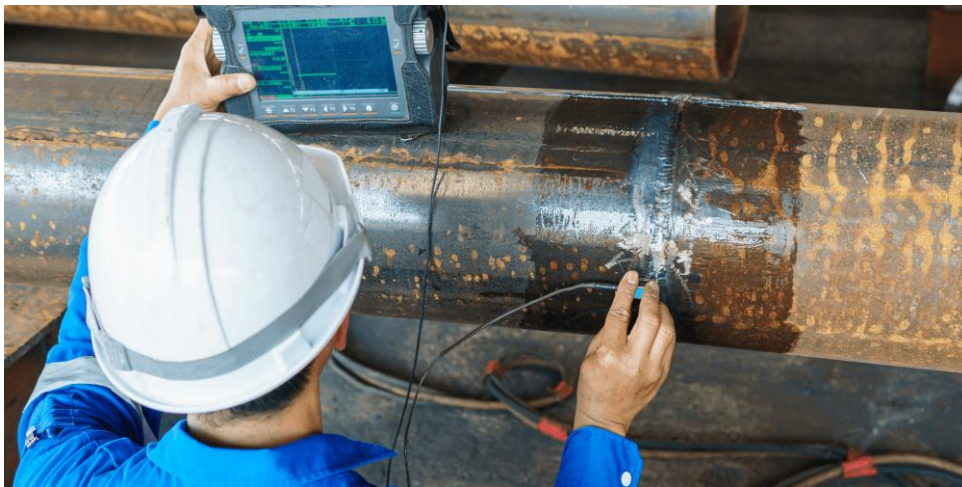
Figure 6 Ultrasonic - NDT - on pipes using an ultrasonic flaw detector (ETITB, 2024)
