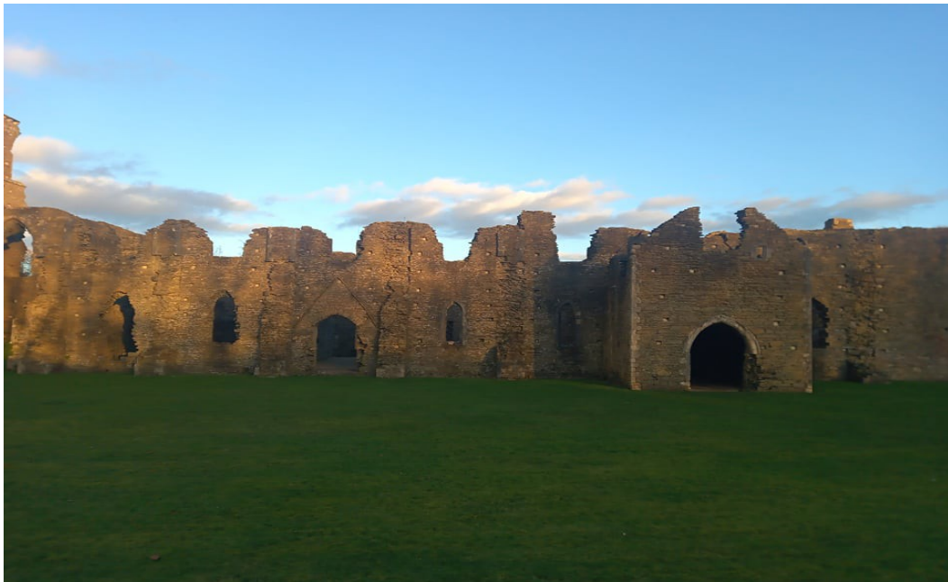
Abbey Ruins – The Oldest Buildings, Front. 5
