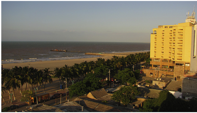
Fig. 5. Example of Urban beach, Riohacha located at La Guajira department (Class V, Litter Grade A).
