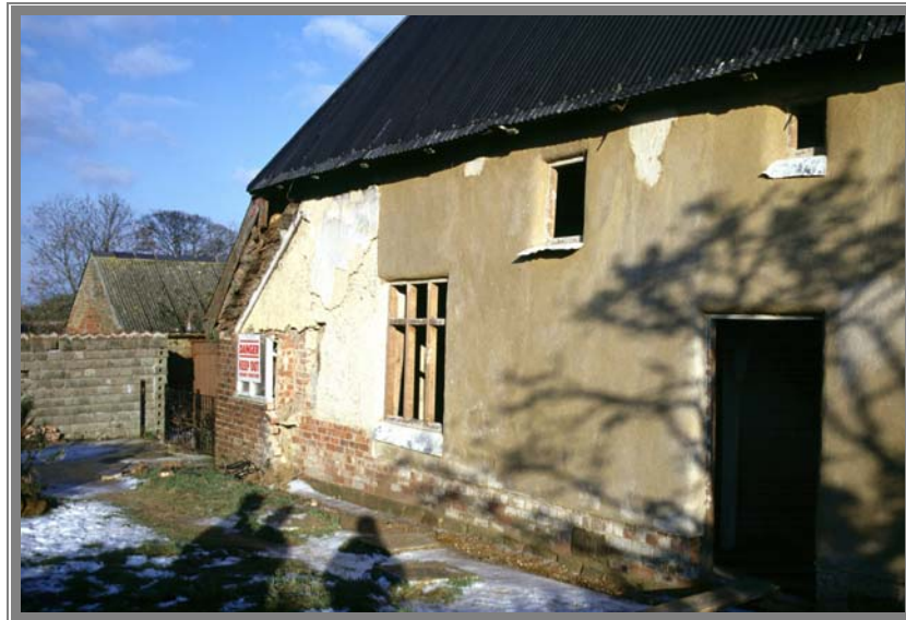
Plate 11 A sensitive refurbishment can exemplify sustainable construction principles if designed and managed appropriately
