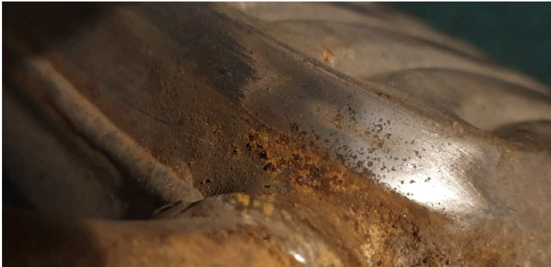
Figure 3: Cleaned steel with pits of dark rust embedded
