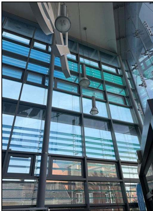
Figure 9 - Site Visit, 15 June 2026 – Lobby Room Office spaces
