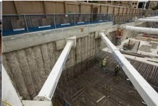
(Braced secant piles) (Bascol.co.uk)
