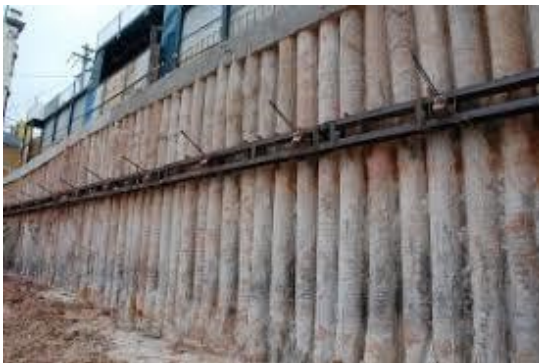
(Anchored secant piles) (Bascol.co.uk)
