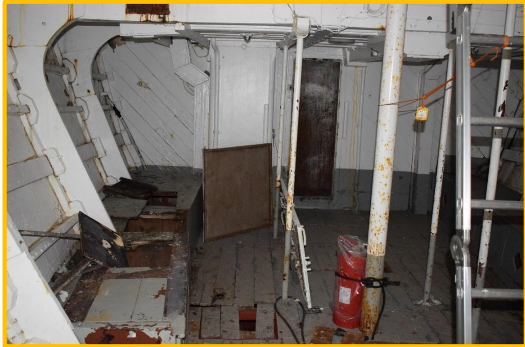
Figure 18: Main accommodation facing aft toward bulkhead 9
