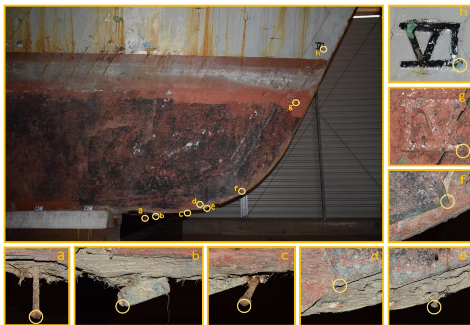
Figure 39: Monitoring points established to record the bow
