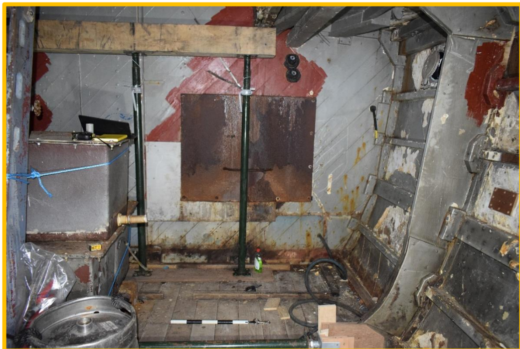
Figure 19 Officers compartment looking aft to the forward face of bulkhead 12
