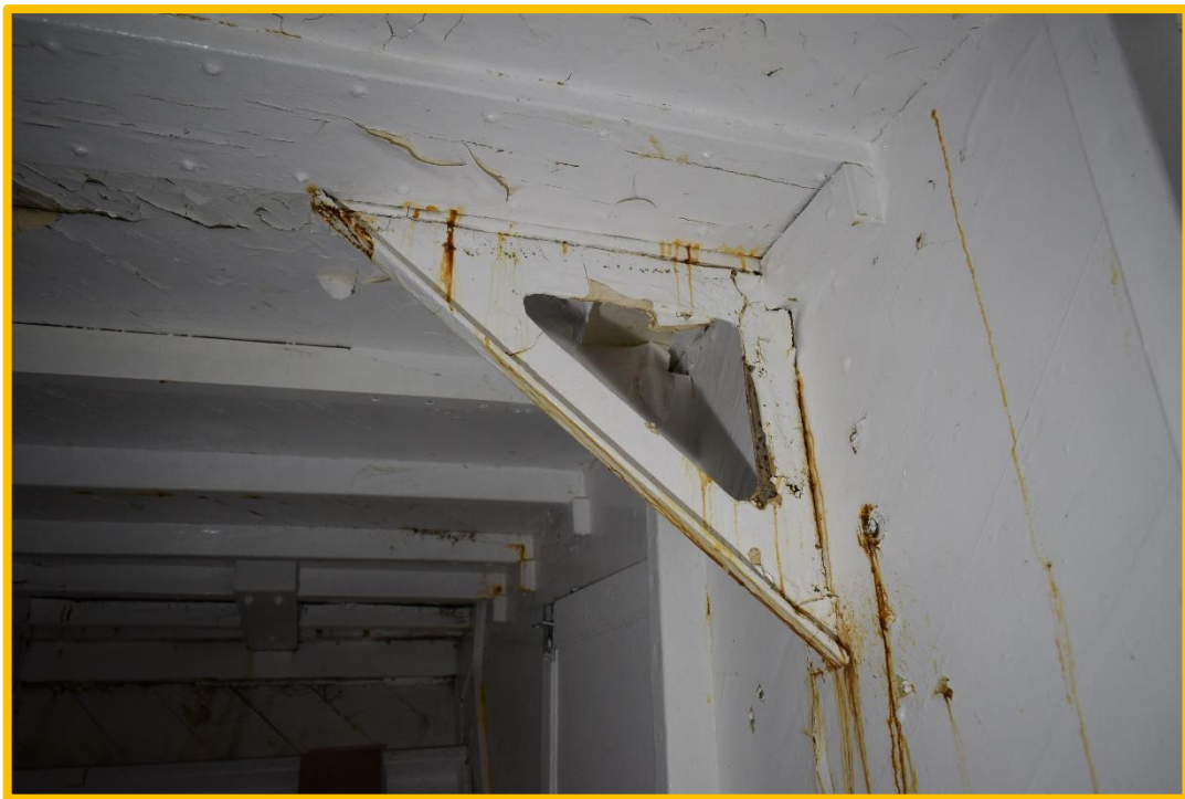
Figure 9 Steel knees added to support mark 1 mine chutes
