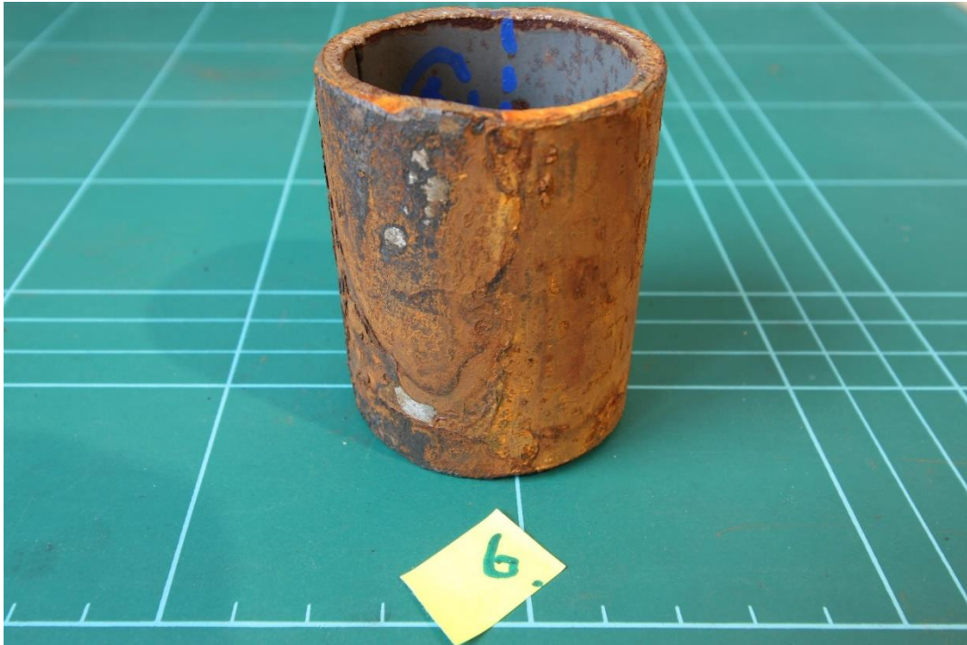
Figure 4.33 Pipe Sample 6 Ambient - Closed-cell elastomer foam insulation – Lower 180°
