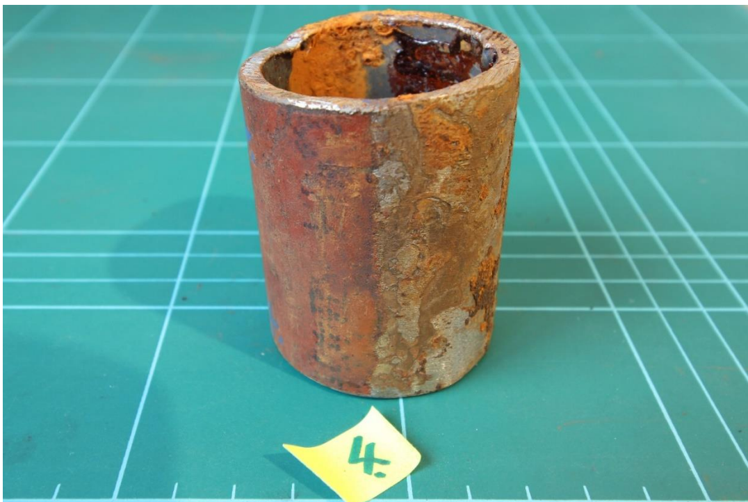
Figure 4.24 Pipe Sample 4 Ambient - Rock Mineral Fibre Insulation - Upper 0°
