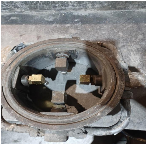
Figure 3:9. Water Head Assembly
