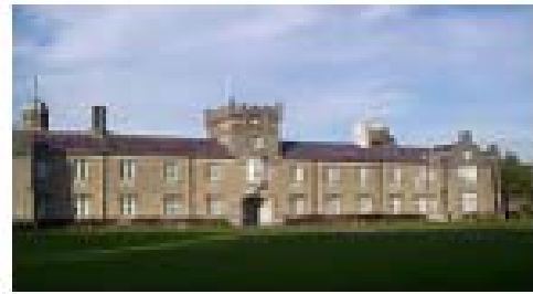
St David's Building current
